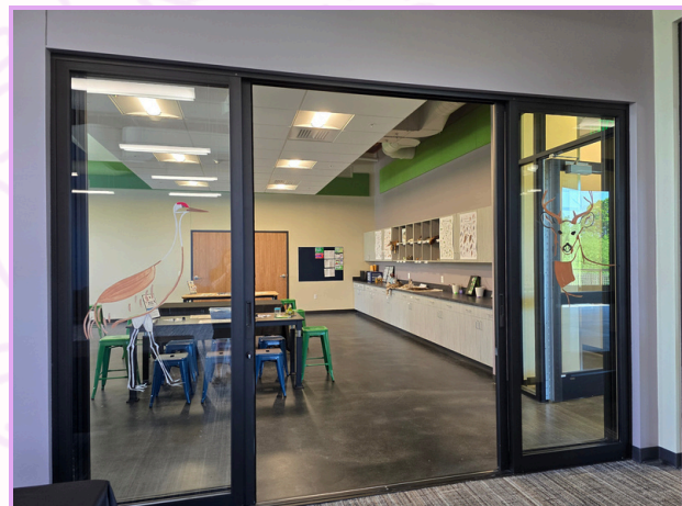
Environmental Education Classroom doors, viewed from the Multi-purpose Room
